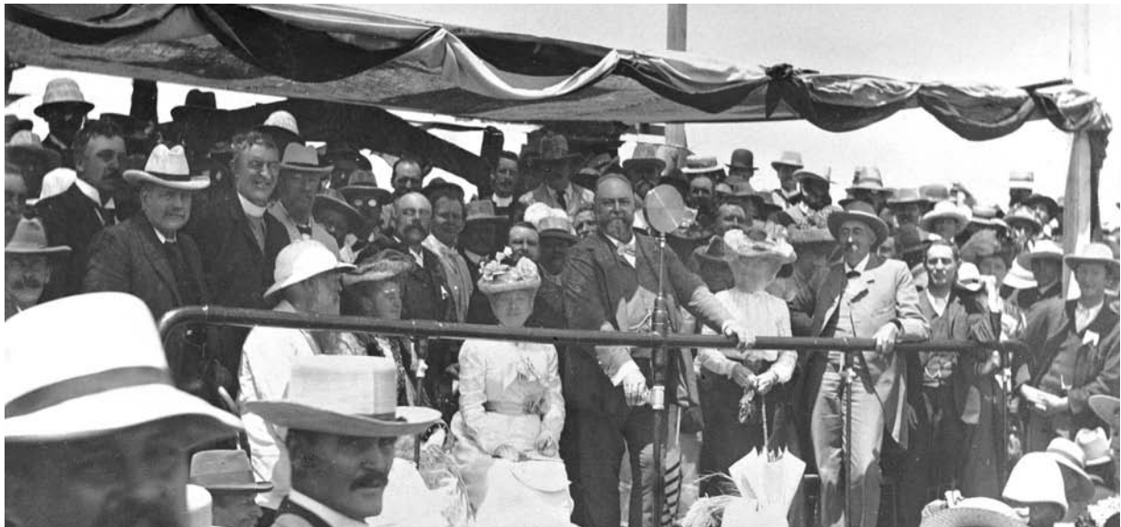
Sir John Forrest officially opens the Scheme by turning on the water at Coolgardie on 24 January 1903.
