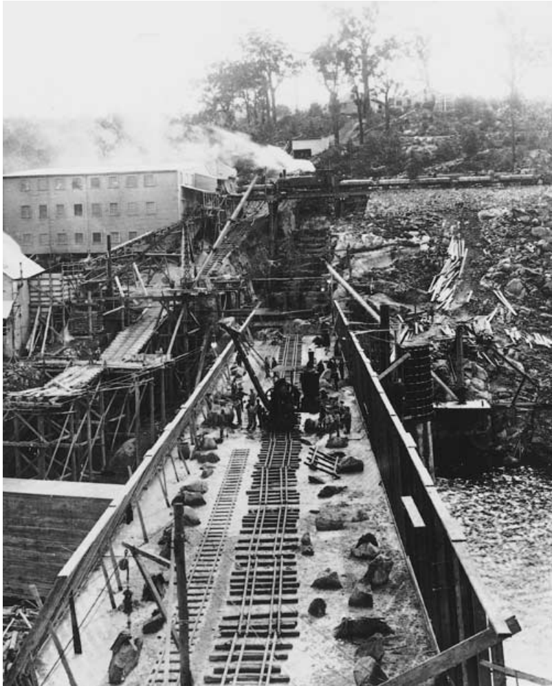
Building the weir wall showing 'plums' in the concrete 1900
